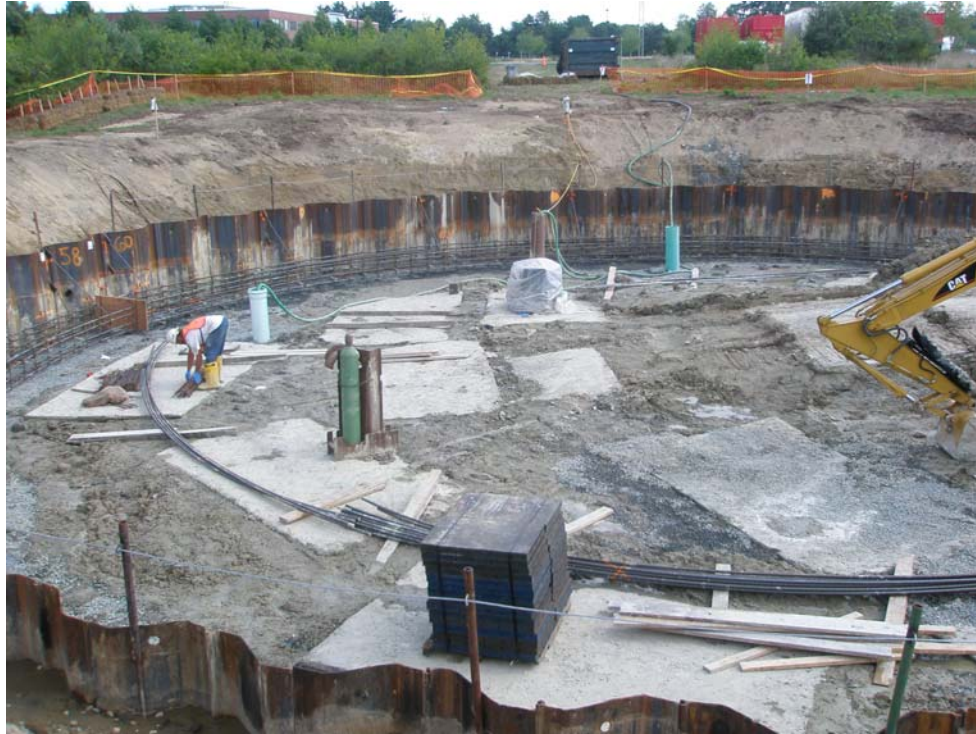
Photograph 1 – Installation of Reinforcing Steel
