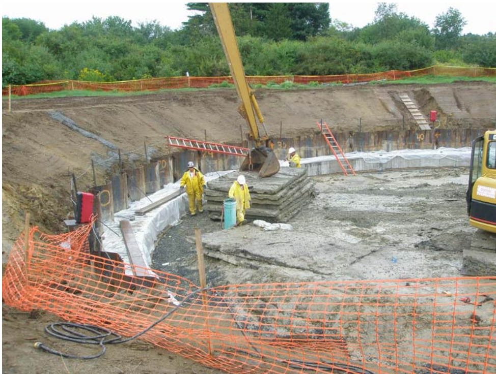
Photograph 6 – Consolidation of Tundra Mats in Preparation for Excavation
