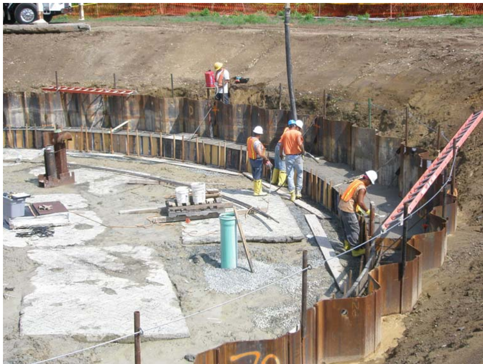
Photograph 4 – Continued Concrete Pouring and Strain Gauge Installation (top center)
