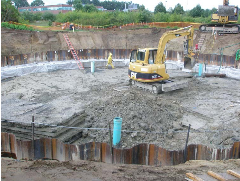
Photograph 5 – Completed Upper Wale
